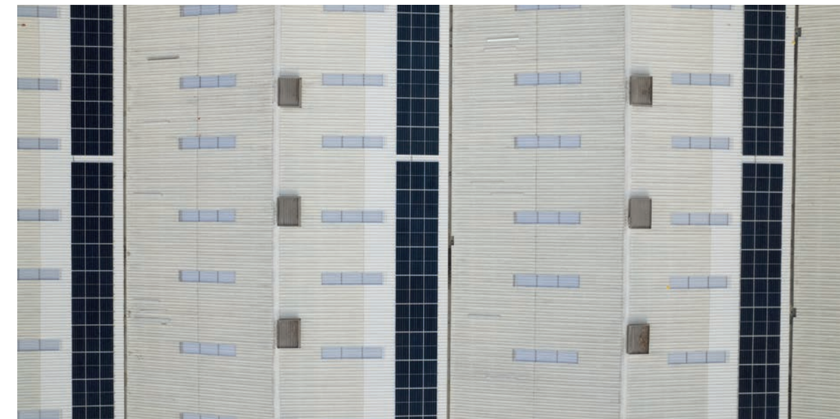
Solar panels on the Adarse logistics asset within Ecogis.
